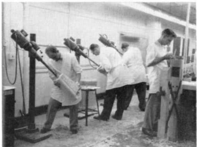
PROSTHETICS EDUCATION AT NYU—Students of the courses in above-knee prosthetics offered by New York University during the 1956-57 academic year engage in shop practice in the construction of the above-knee prosthesis
