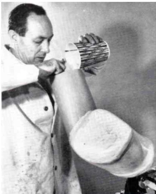
Fig. 17. Pouring polyurethane foam into cardboard form.
