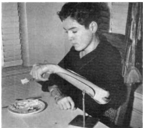
Fig. 4. The stand feeder of March 1945. The aluminum base permitted the patient to move the feeder horizontally across the lapboard by body movements for best position.
