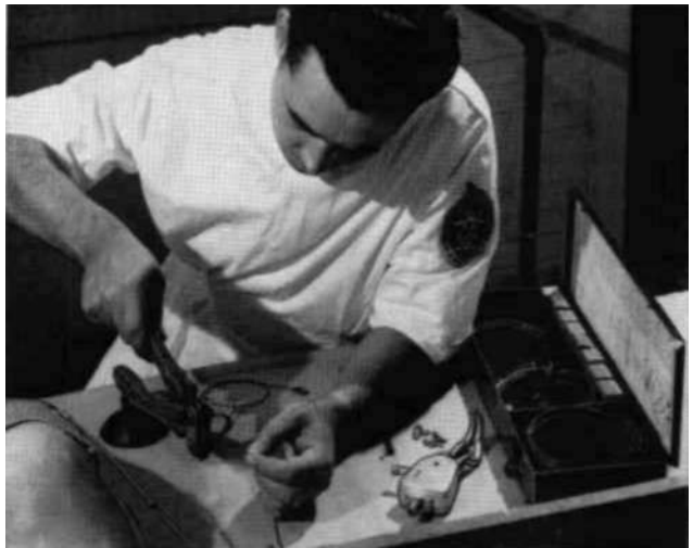
IMPROVED CABLE-TRANSMISSION SYSTEM—Anton Leins, Jr., formerly Orthopedic Technologist with the Veterans Administration Prosthetics Center, New York City, demonstrates use of the hand swage supplied with the new ACCO-APRL prosthetics kit. Swaging cold-fuses the terminal connections to the cable to form an attachment as strong as the cable itself. Besides the swaging tool, the kit contains enough parts to provide control systems for about 30 complete arms.
