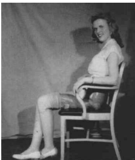
Fig. 32. Method of preventing excessive hip flexion during sitting. Normal shank restrains artificial shank.
