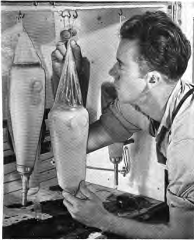
Fig. 29. Forearm and upper-cuff sections in curing oven.
