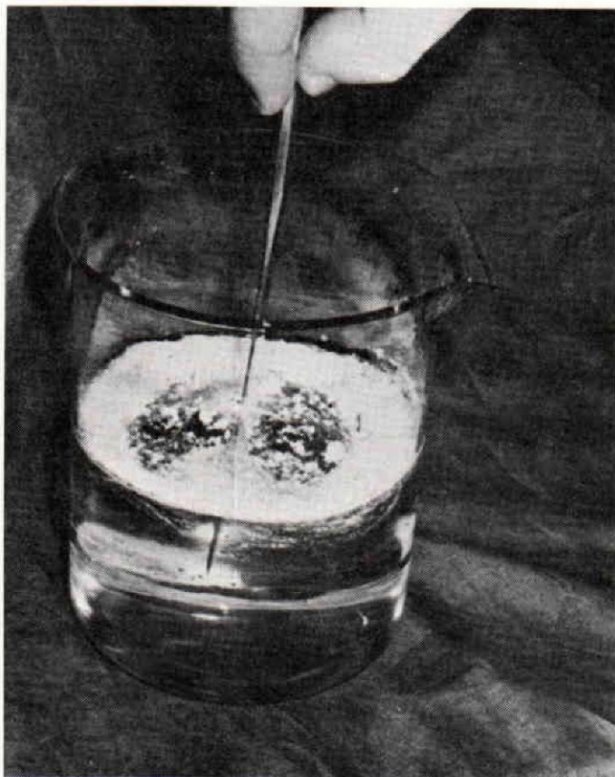
FIGURE 15.—Stirring of catalyst into methyl methacrylate.
