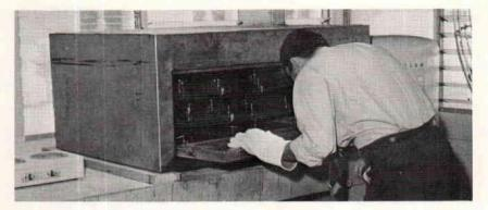
Heat the  $\frac{3}{8}$ -in. material for 36 hours at 275-300 deg. F. to drive out the moisture absorbed by the polycarbonate. If the water is not removed the resulting socket will contain bubbles. It must be maintained at a temperature well below the melting point. A pizza oven was used quite satisfactorily in the development program.
