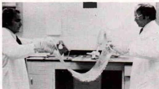
Fig. 1. The heated polypropylene sheet is lifted slowly from the oven.
