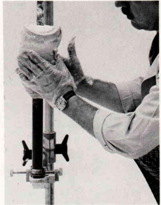
Fig. 7. Impregnating the stockinette with polyester resin and silica powder.
