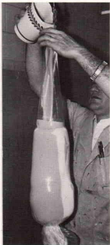
Fig. 7. The outer PVA bag is in place and the resin is being poured.
