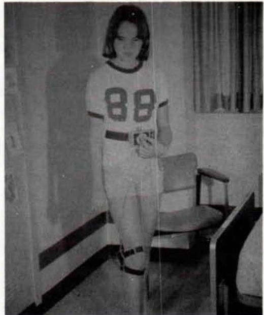
Fig. 19. Patient with peroneal functional electrical stimulation device in place. The electrodes in this case are external to the body.
