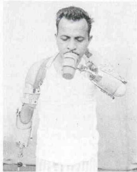
Figure 2. Bilateral amputee, drinking water, holding tumbler with the help of tumbler holder; wearing tweezer on the other side.
